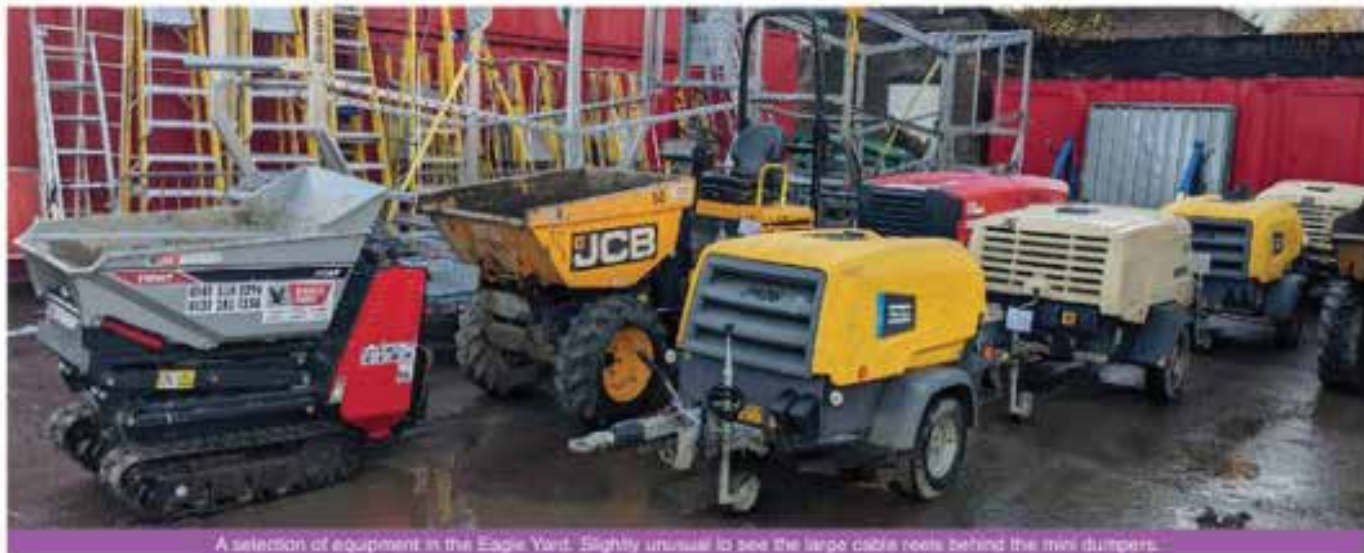
A selection of equipment in the Eagle Yard. Slightly unusual to see the large cable reels behind the mini dumpers.
